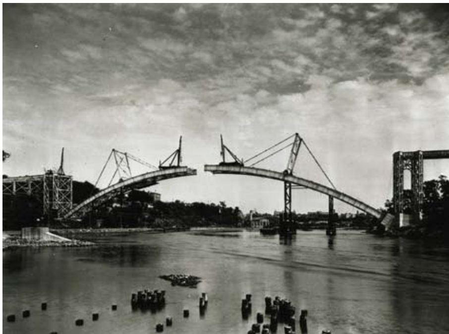
Fig. 38 The Henry Hudson Bridge under construction , June 19, 1936 Courtesy of MTA Bridge and Tunnels Special Archive Photography: Richard Averill Smith
